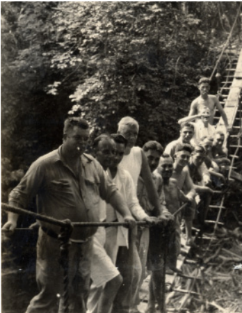
A suspension bridge over the Rio Grande River at Camp Deakne, constructed by the battalion's Company A.
